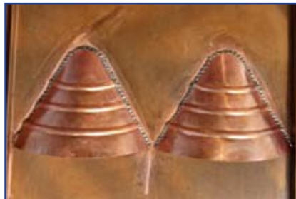
Covers for Vents to level the air pressure and reduce condensation
