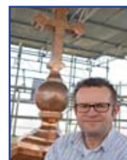
Simon aloft, by the cross on the top of the dome, then protected by scaffolding.
